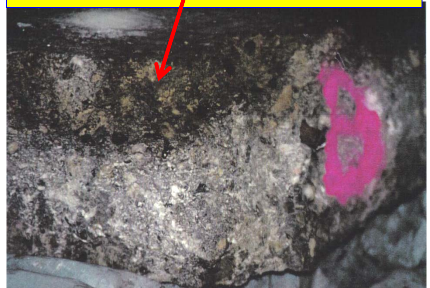
Side View Of Concrete Permeated With Oil-Note the oil has penetrated to depth of 2 to 3 inches
